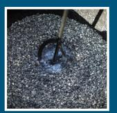
2. Mix EASIHOLD with your stones until they are evenly coated. You can mix using a mixing paddle, or simply by shaking and rotating the stones using a gauging trowel until fully coated throughout.
