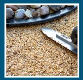
4. Compact the stones using a trowel, or by standing on wooden planks. A flat surface will be a lot more robust than with protruding stones when subjected to foot traffic.
